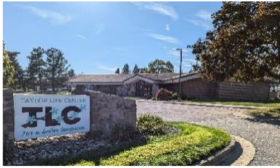
Mason – Administrative Office and Outpatient Clinic
