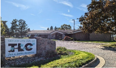
Mason – Administrative Office and Outpatient Clinic
